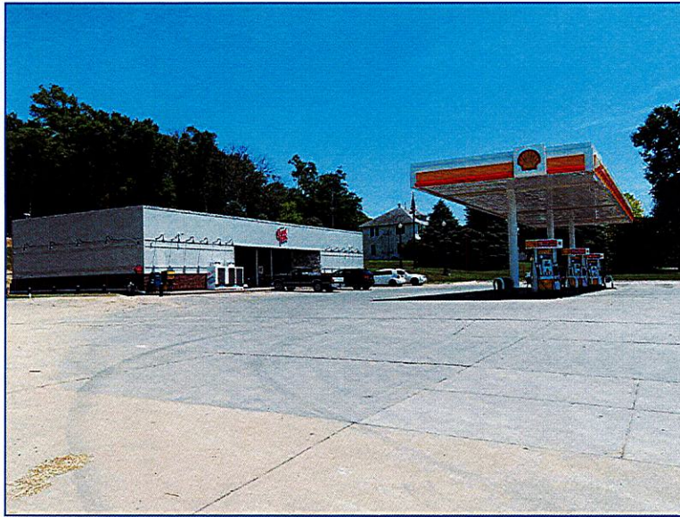
14151 WABASH AVE, TAYLOR OIL COMPANY INC, 1 06/25/2020
