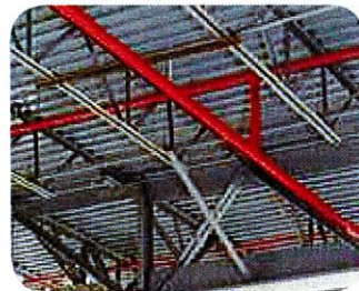
Continuous Truss with Transbay
